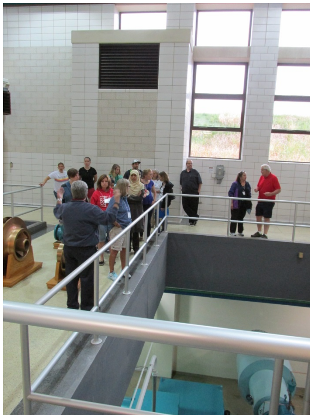
McGhee explaining how water is pumped from the reservoir
