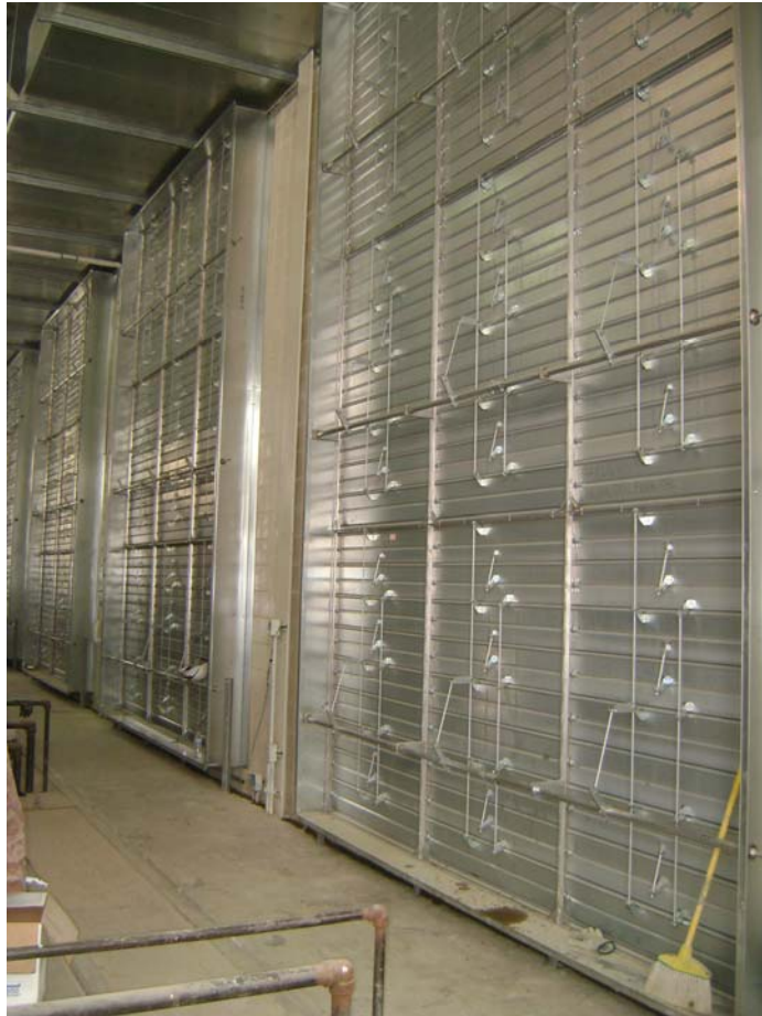
Generator Exhaust Louver Progress
