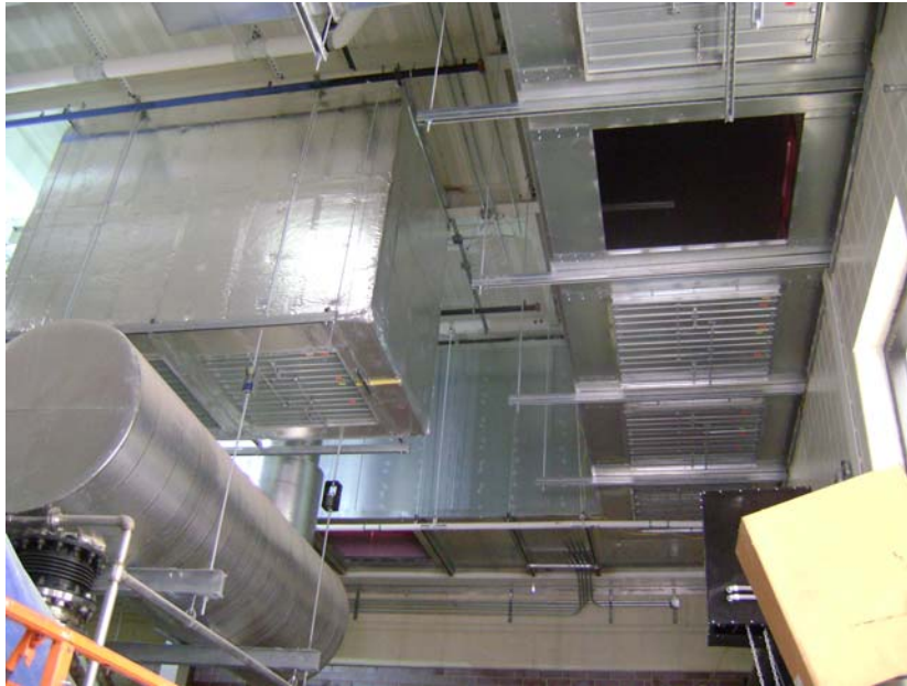
Generator Building Ductwork Progress
