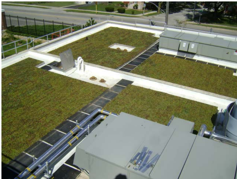
Vegetative Green Roof Progress
