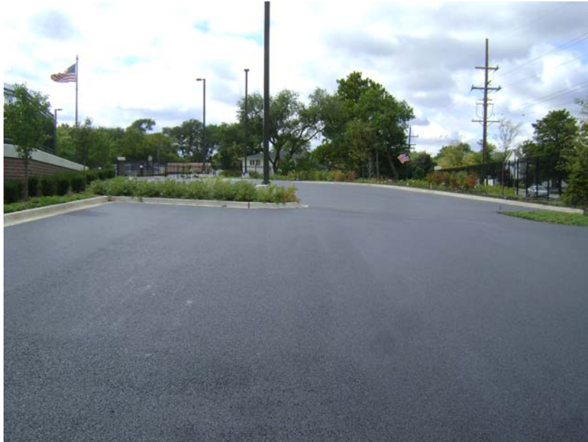
Parking Lot Pavement Completion
