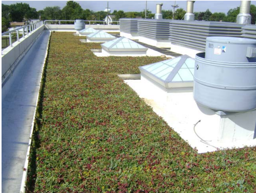
Vegetative Green Roof Progress
