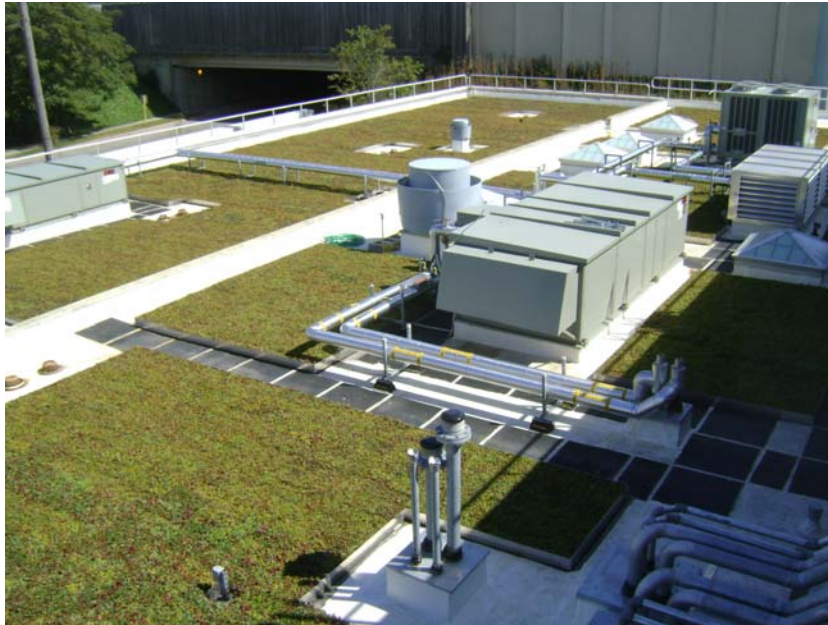
Vegetative Green Roof Progress
