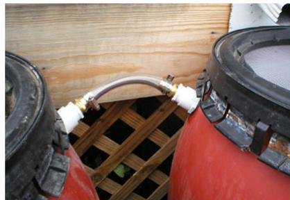
There are many ways to connect one barrel to another. Here, we used some plastic tubing and hose clamps.
