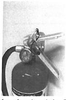
In addition to annual maintenance checks by the service company, employers are required to inspect them monthly. The back of the tag on the extinguisher is set up for the date and initials of the person conducting the inspection.
